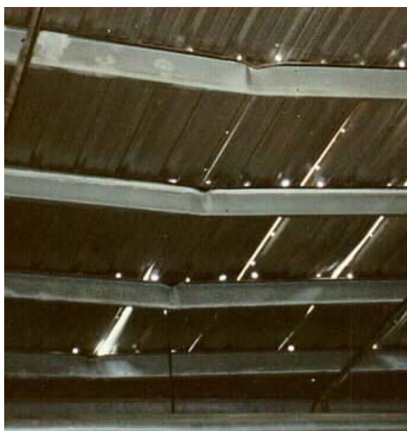
Figure 6-3 Local Buckling in Maximum Moment Region of Cold-Formed Beams and Panels
