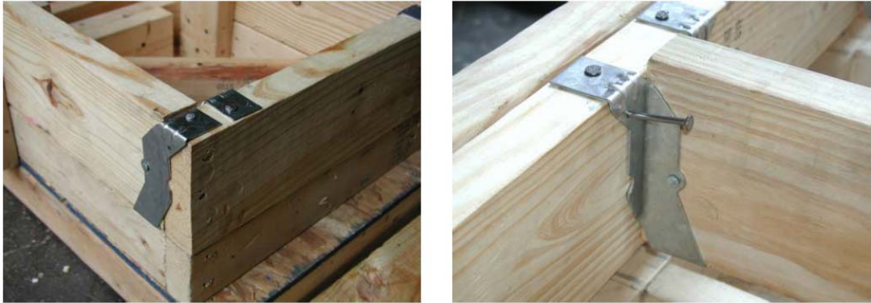
Figure 8-3 Wood Stud Hanger Connections
