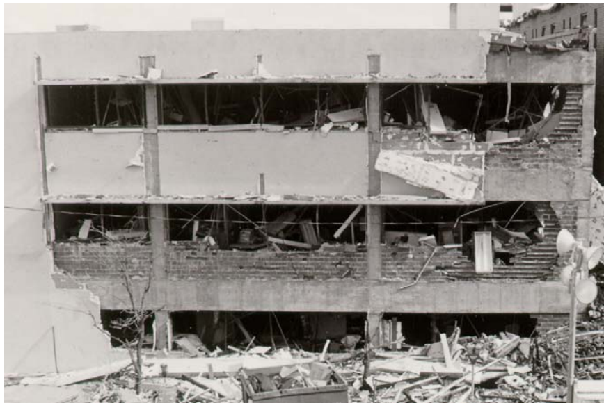
Figure 41. Portion of Reinforced Concrete Frame Building Near Oklahoma City Bombing with Cladding Failure
