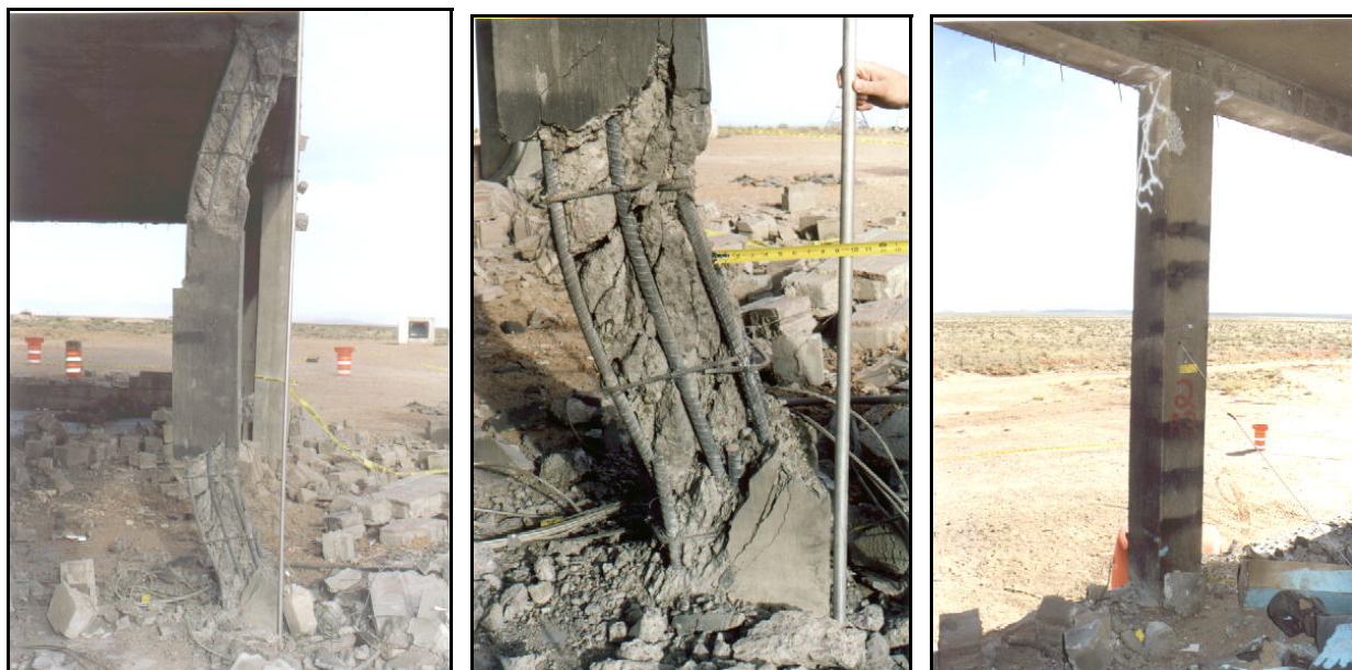
Overall View of Failed Column Bottom of Failed Column Damaged Second Floor Column
