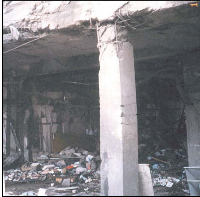
Figure 43. Damage to Concrete Column at 5 m from South Quay IRA Bombing in London
