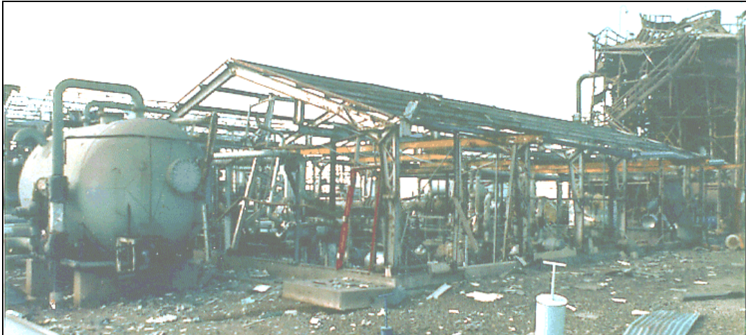
Figure 46. Typical Pre-Engineered Steel Building and Multi-Story Steel Frame Building (in Background) with Cladding Failure Caused by Blast Loads
