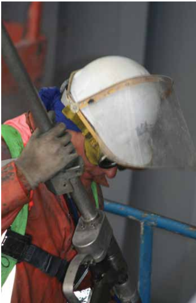
Above, clockwise from left: A DRAA Spillway gate contractor prepares to power wash one of the gates in preparation for inspecting and painting of the gate.; A DRAA contractor inspects and notates findings during a bridge inspection at Big Bend Dam power house; Kathlene (Katie) Shook, Omaha District structural engineer and certified bridge inspector, gets a close-up view of the Power house bridge at Big Bend during a required inspection. All photos by Cheryl Moore.
