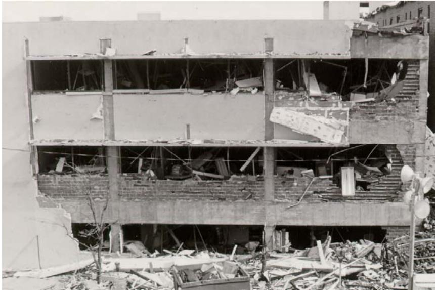
**Figure 44. Portion of Reinforced Concrete Frame Building Near Oklahoma City Bombing with Cladding Failure**
