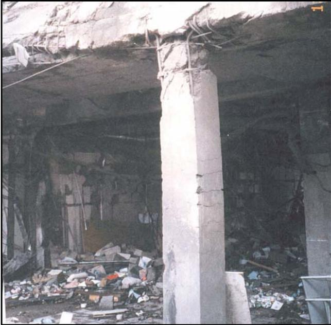
Figure 46. Damage to Concrete Column at 5 m from South Quay IRA Bombing in London
