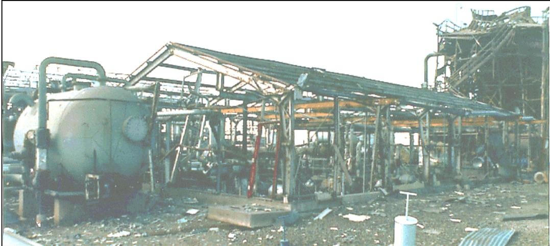
**Figure 49. Typical Pre-Engineered Steel Building and Multi-Story Steel Frame Building (in Background) with Cladding Failure Caused by Blast Loads**
