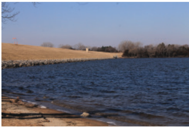
One of the dams that will soon be undergoing a periodic Dam Safety Inspection is Salt Creek Dam Site 8 at Wagon Train Lake near Hickman, Nebraska. (Photo by Eileen Williamson)
