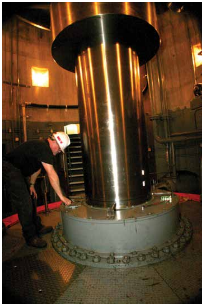
Senior Mechanic Rod Bergin inspects a hydro-electrical generator's turbine shaft during annual maintenance of the unit at Fort Randall Dam. (Photo by Al Barrus)
