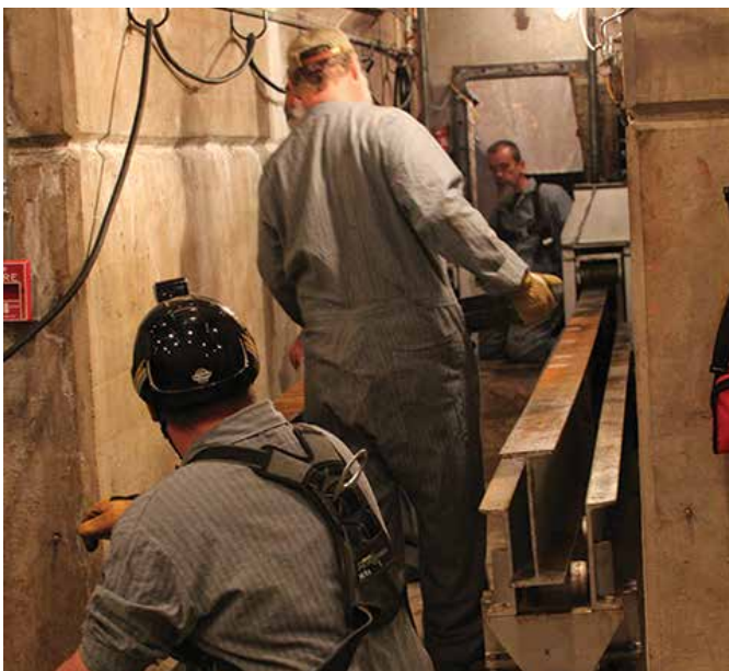
Project crew members, Dave Timmerman, Steve Neumann and Mike Schnetzer, carry scaffolding platform sections for placement in the draft tube. Photo by Karla Zeutenhorst, Natural Resource Specialist.
