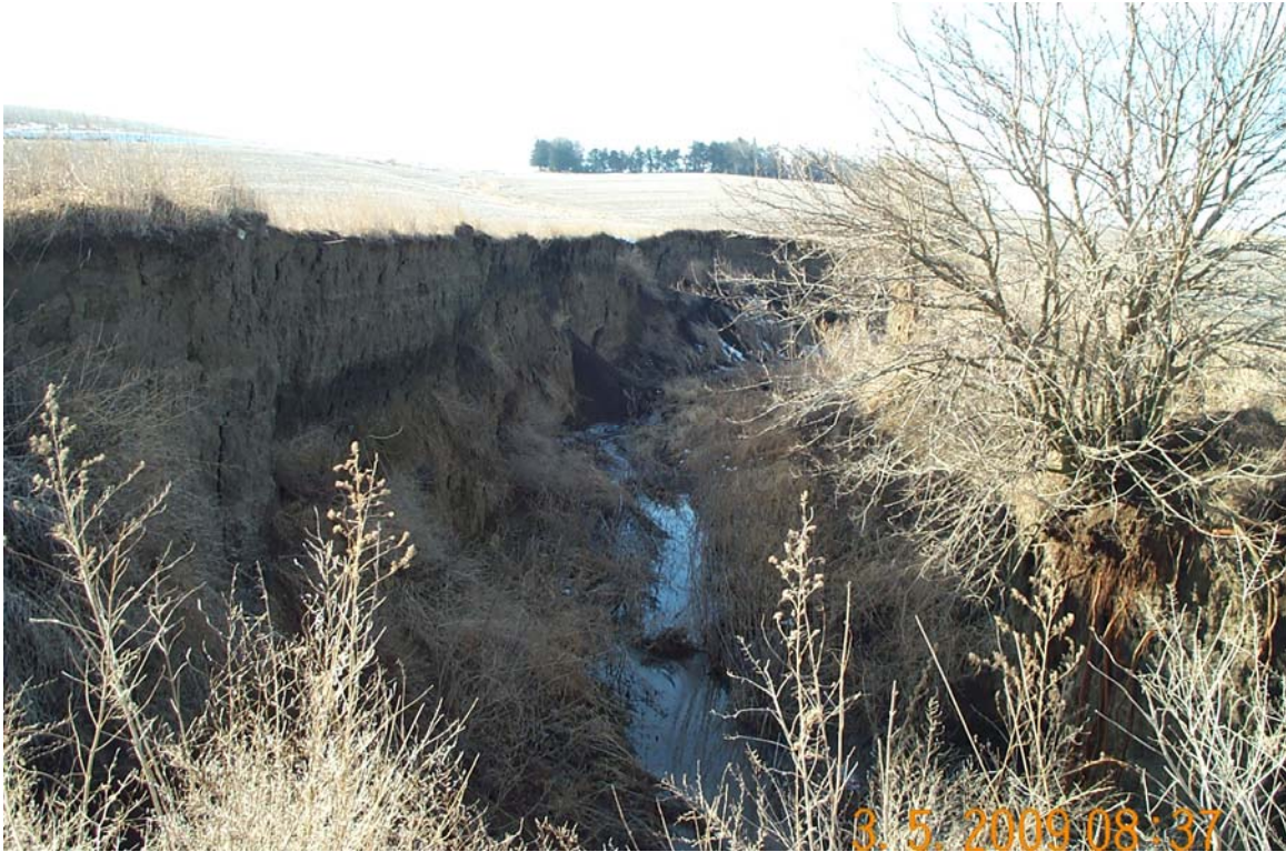
#1 Looking North from A Road bridge
