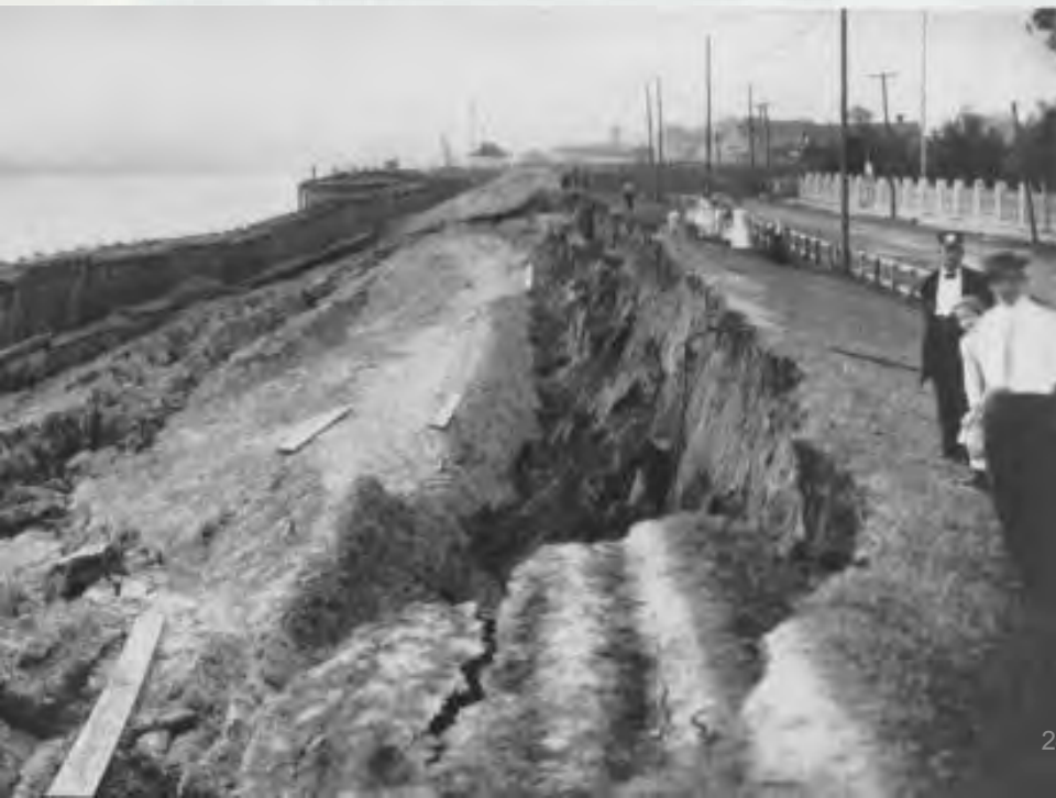
Riverside Slope Failure *Most Common
