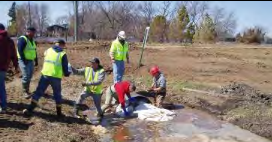
Emergency closure of culvert
