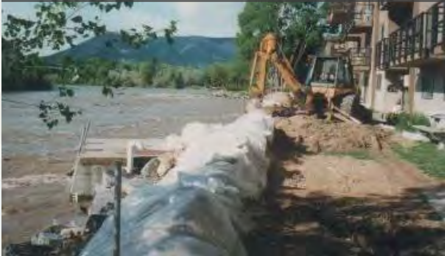
Sandbags to Earthen Levee
