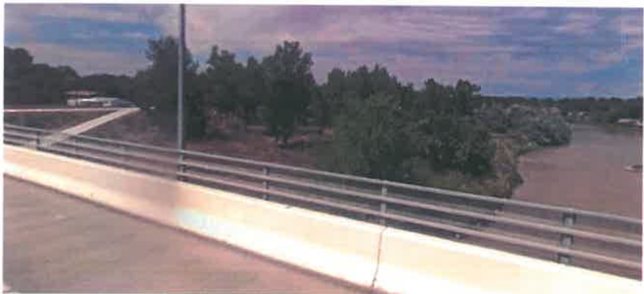
Figure 15. Greybull Levee (to the left under the white bike path) as seen from the Greybull Avenue Bridge, Looking Upstream
