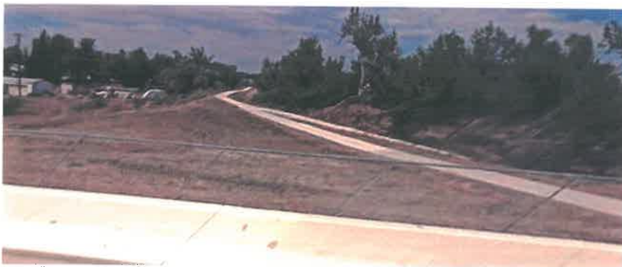
Figure 16. Greybull Levee Adjacent to Residences as seen from Greybull Avenue Bridge, Looking Upstream
