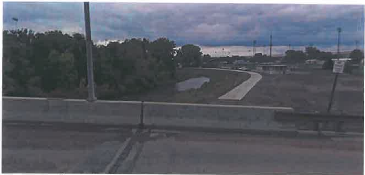
Figure 19. Sheridan Levee with Bike Path as seen from the East 11th Street Bridge
