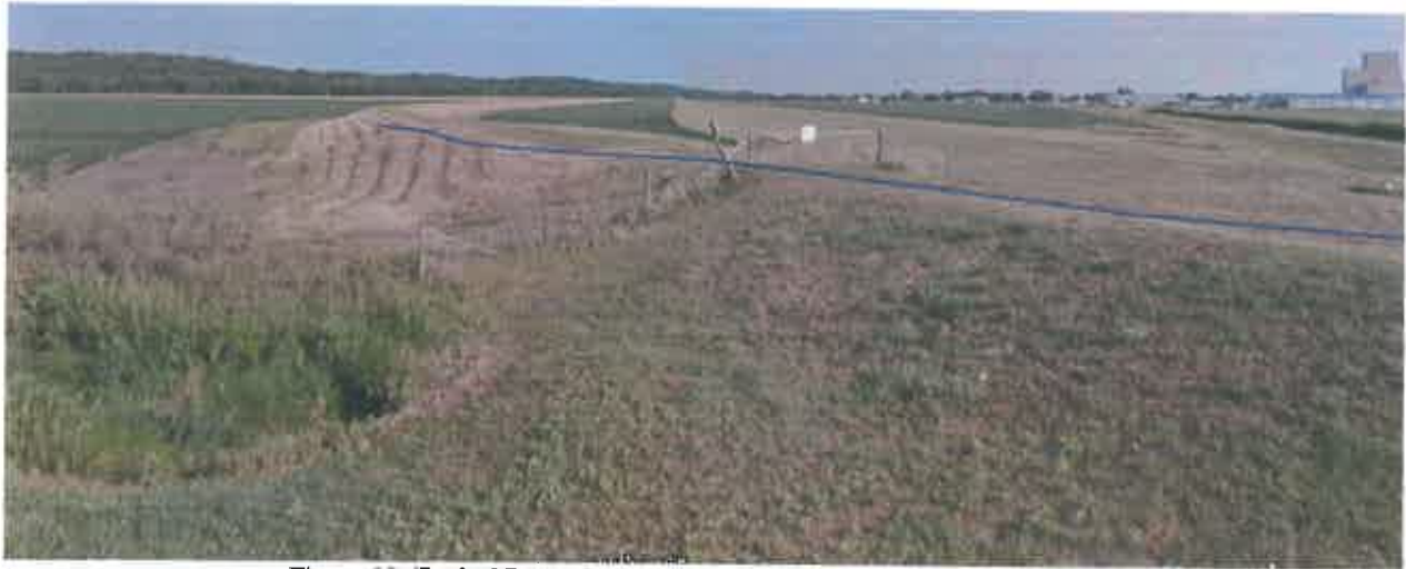
Figure 22. Typical Levee Section (Blue Line) as seen from Waters Road
