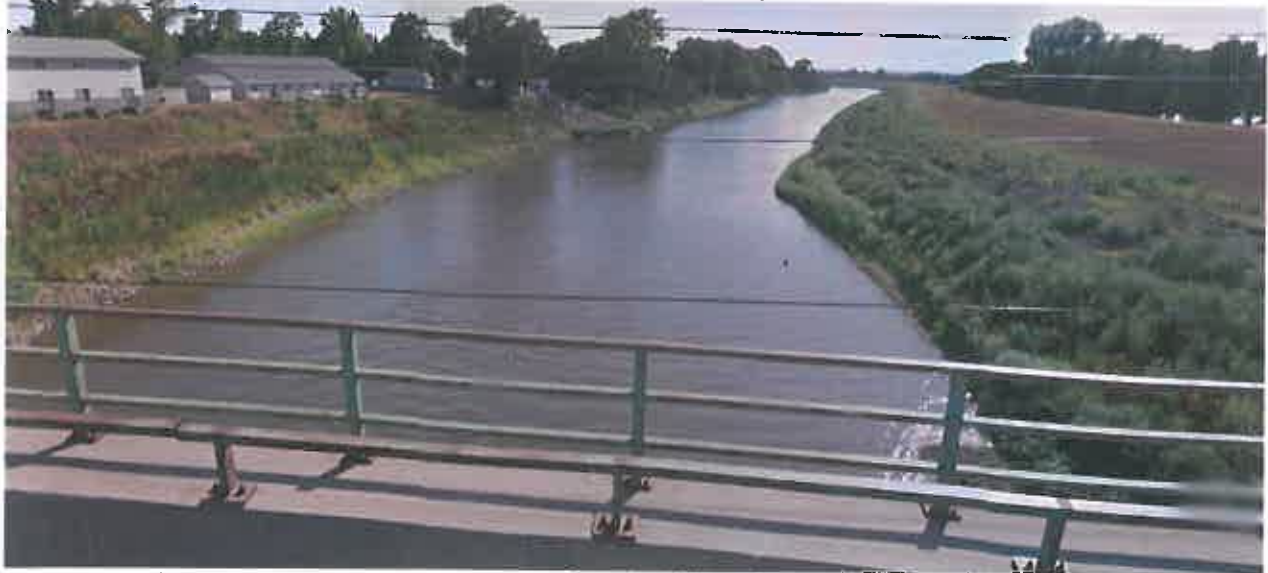
Figure 21. Typical Levee Section as seen from the Military Road Bridge, Looking Downstream
