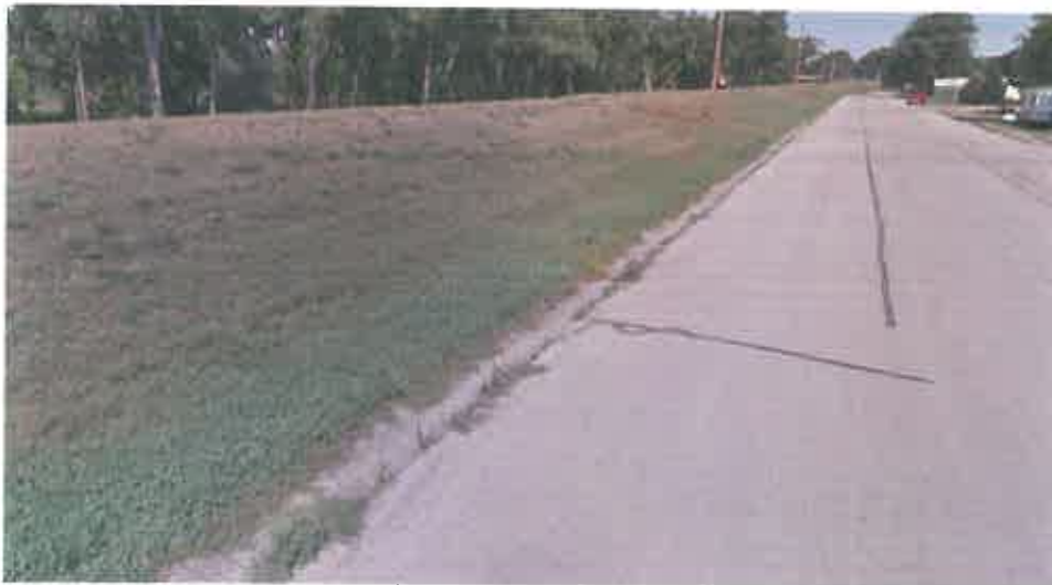
Figure 37. Earthen Levee along Belle Fourche as seen from Edmunds Street
