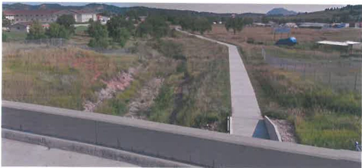
Figure 46. Leveed Section of Deadman Gulch at Interstate 90, Looking Upstream
