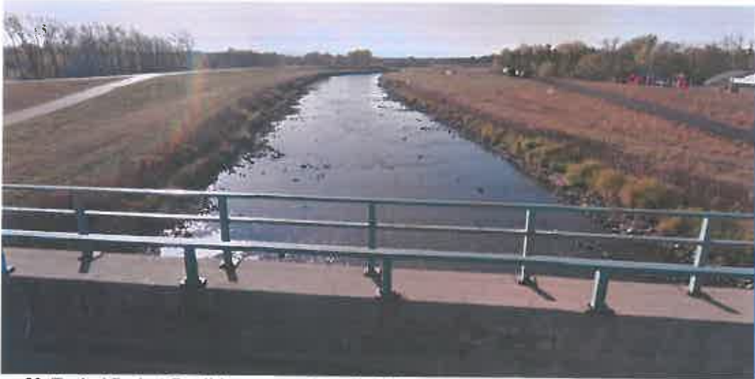
Figure 30. Typical Project Conditions as seen from the 49th Avenue Bridge (South City), Looking Downstream
