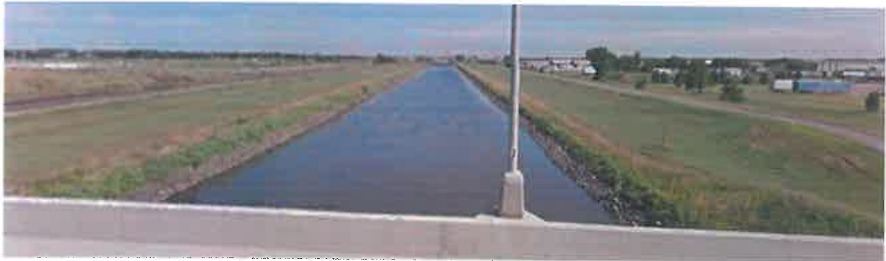
Figure 31. Typical Project Conditions as seen from the East Benson Road Bridge (North City), Looking Upstream
