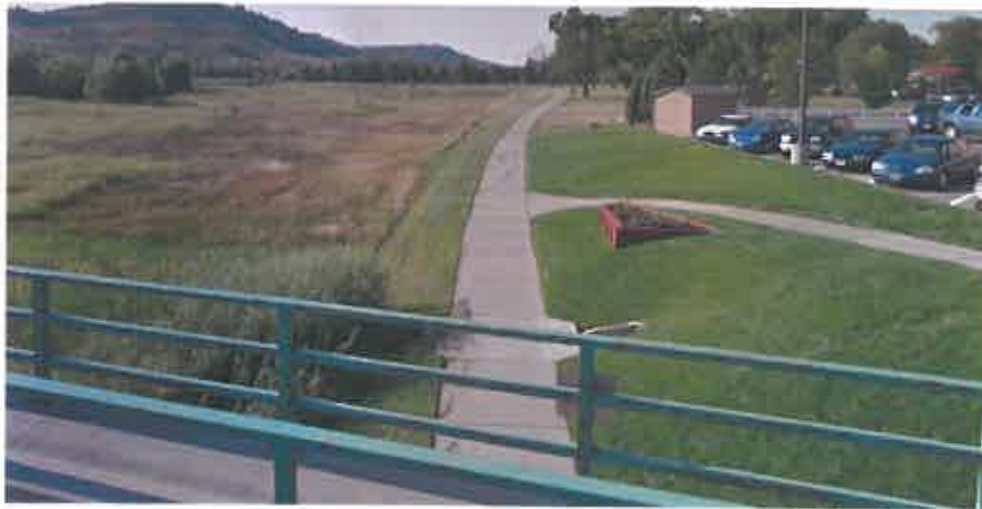
Figure 39. Rapid City Earthen Levee as seen from West Main Street, Looking South
