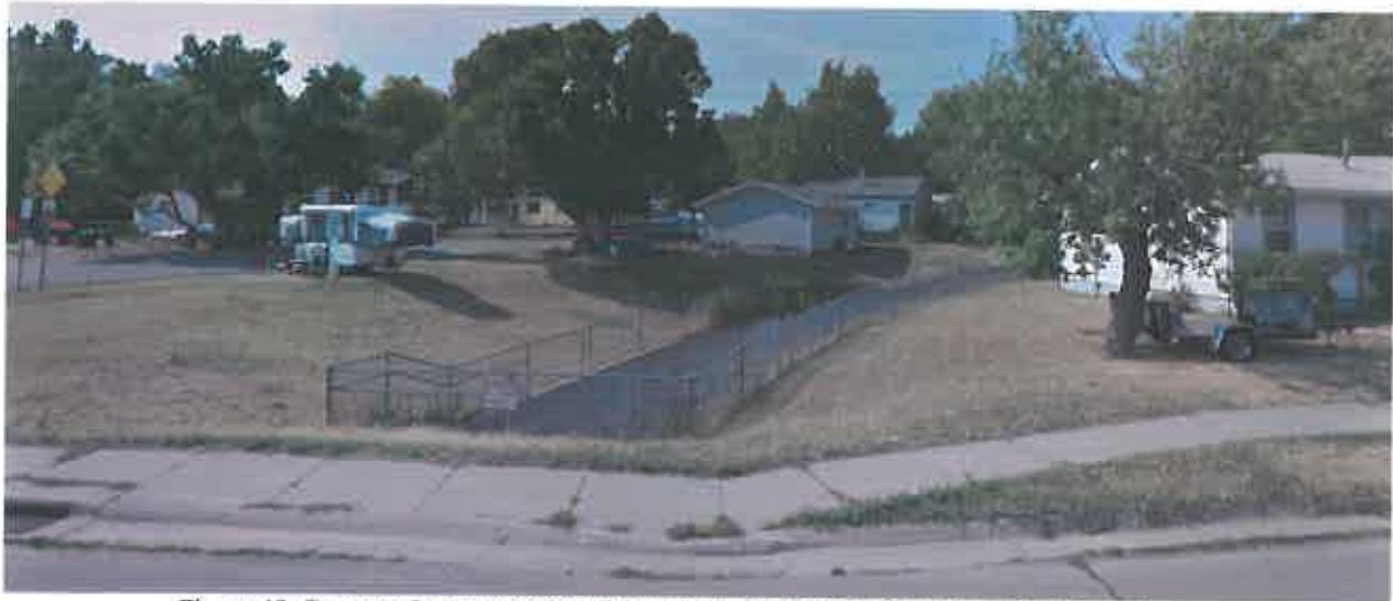
Figure 45. Concrete Improved Channel as seen from Douglas Street, Looking Downstream
