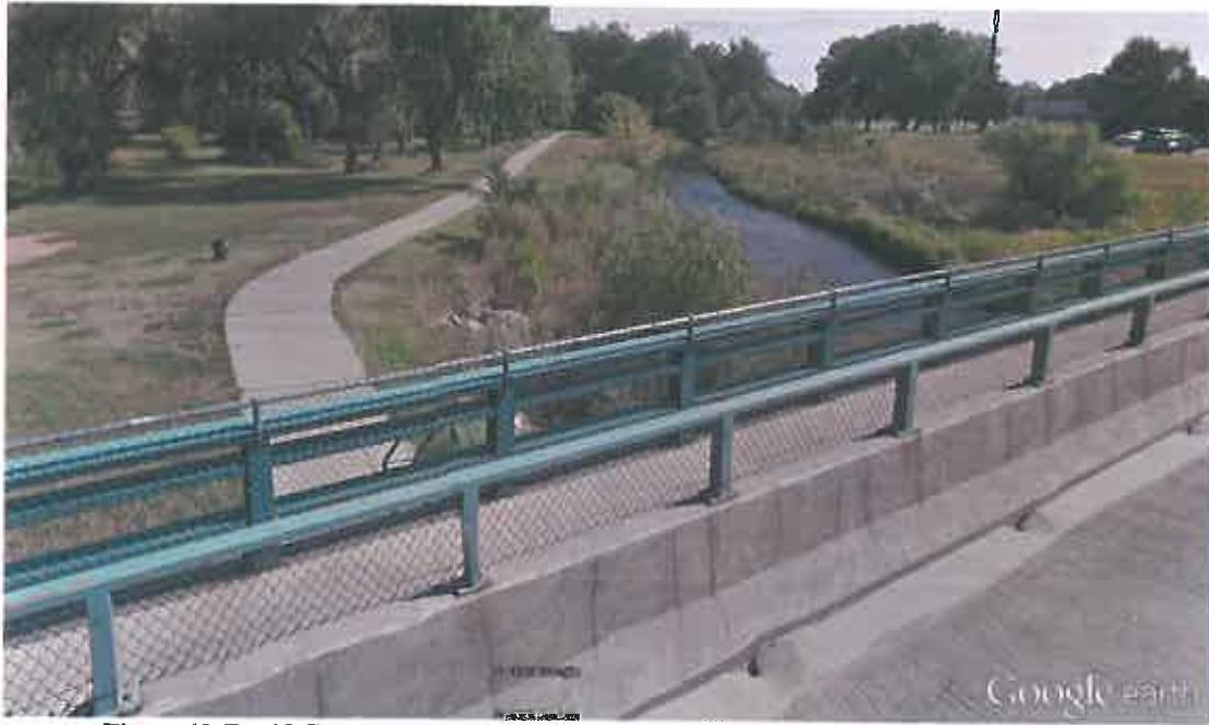
Figure 40. Rapid Creek as seen from the West Chicago Street Bridge, Looking Upstream
