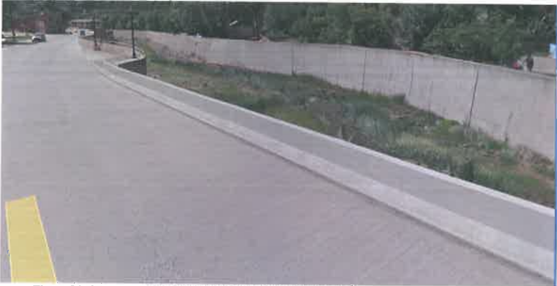
Figure 34. Concrete Floodwall as seen from the North River Street Bridge, Looking Downstream
