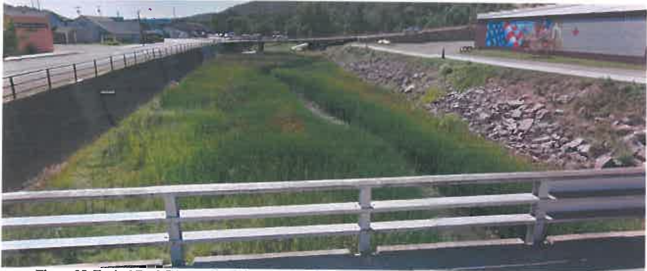
Figure 35. Typical Rock Riprap Conditions as seen from the Jennings Avenue Bridge, Looking Downstream
