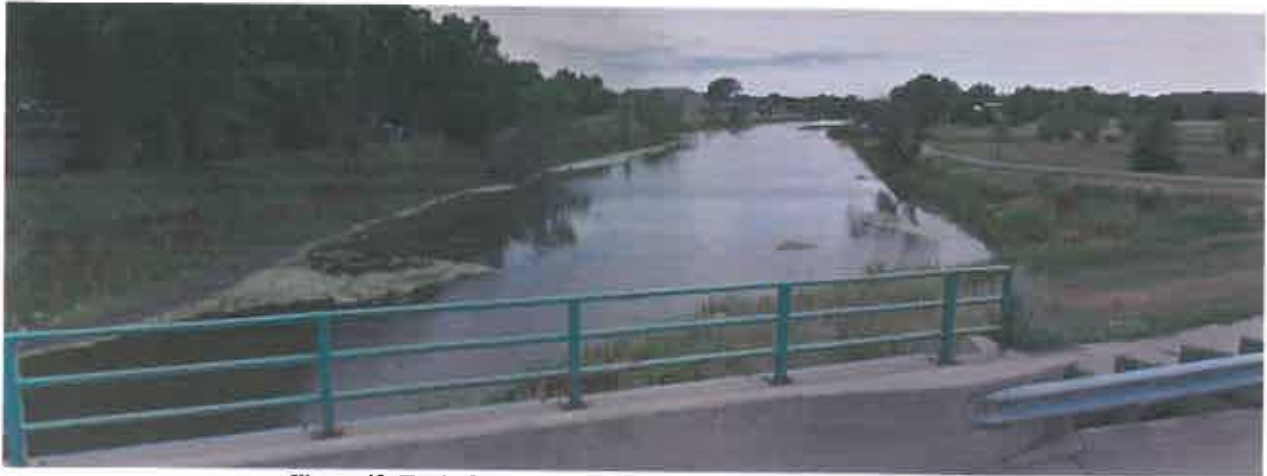
Figure 42. Typical Levee Conditions along Aberdeen as seen from the Milwaukee Avenue Southeast Bridge, Looking Downstream
