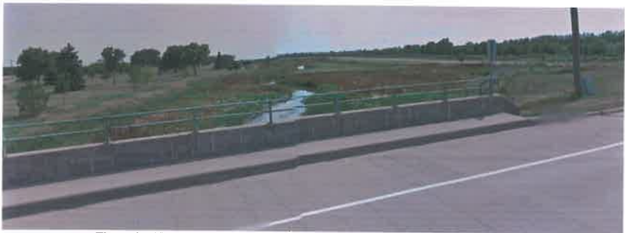
Figure 43. Aberdeen Levee as seen from East Melgaard Road, Looking Downstream
