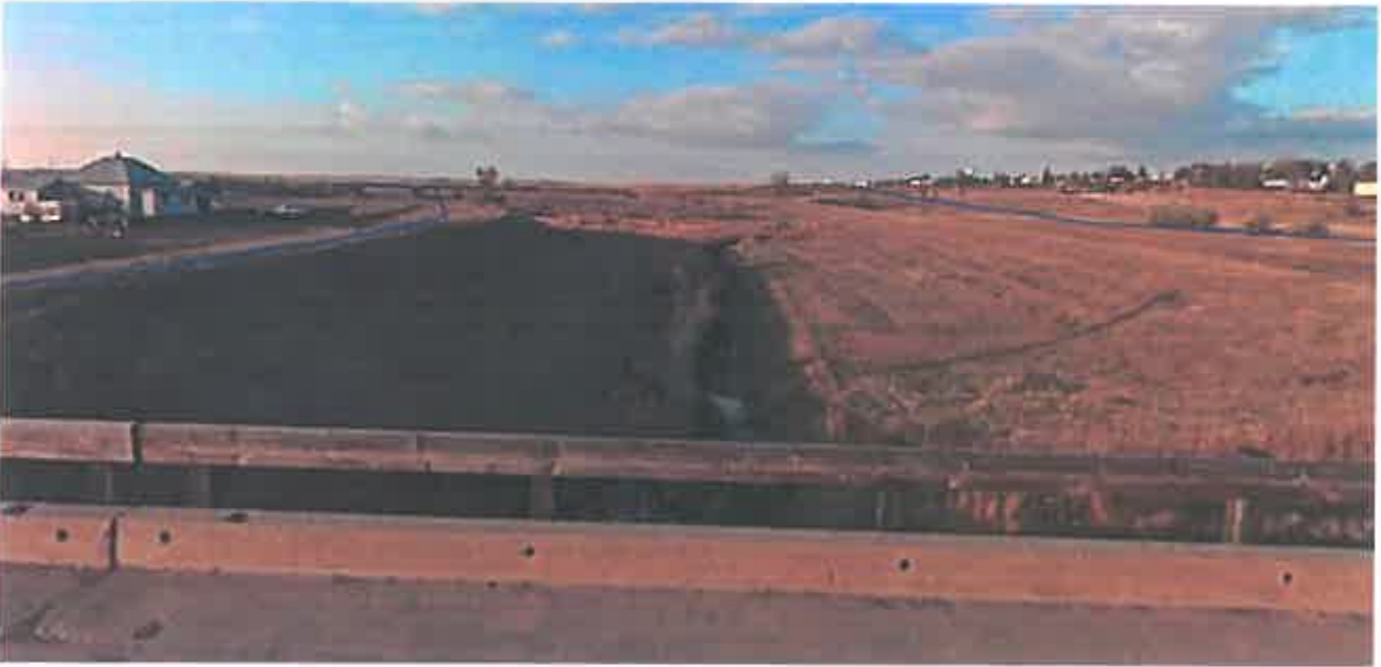
Figure 12. Typical Levees (Blue Lines) along Buffalo Creek as seen from the Hamilton Street Bridge, Looking Upstream
