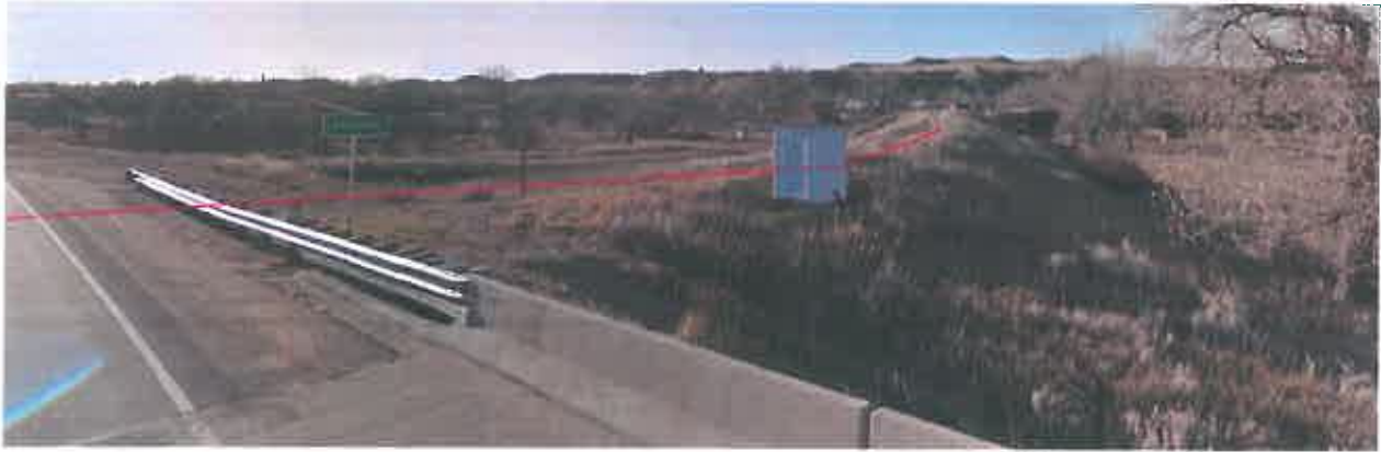
Figure 14. Typical Levee Section (Red Line) at Marmarth as seen from the Highway 12 Bridge
