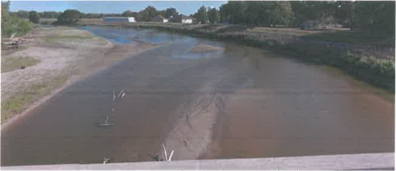
Figure 89. Bridge Street Bridge looking downstream at the Elkhorn River
