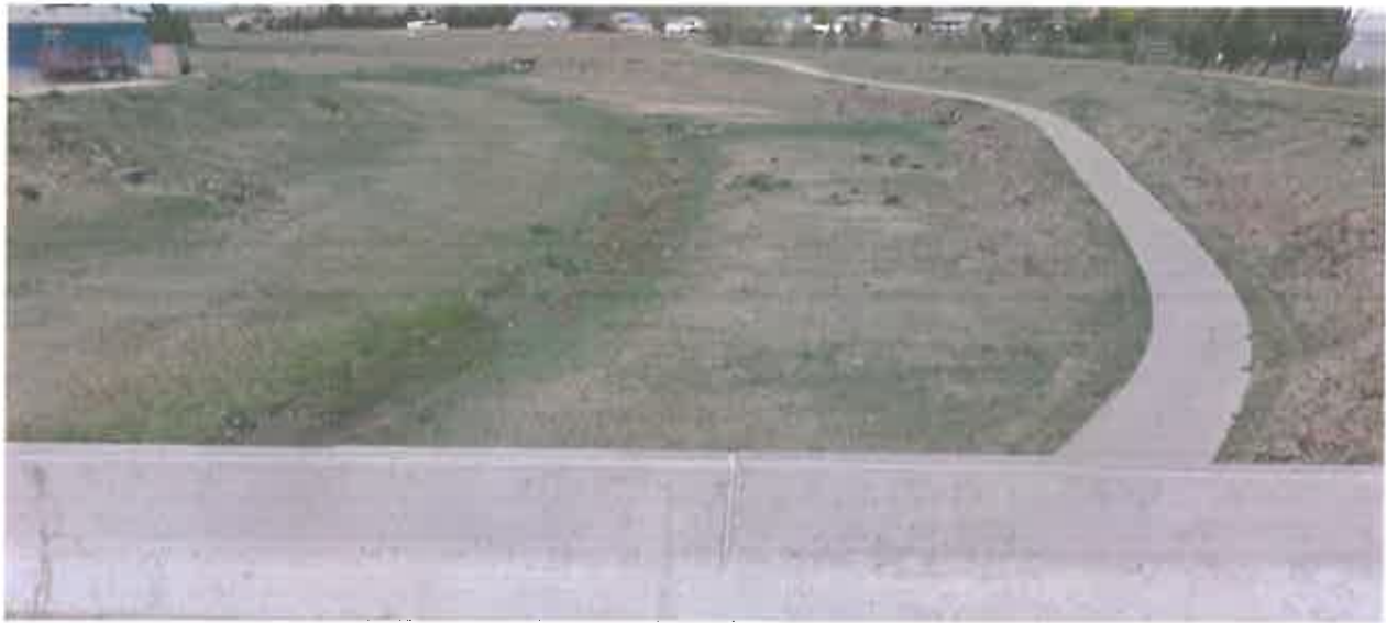
Figure 86. Sidney Draw Road Bridge looking downstream
