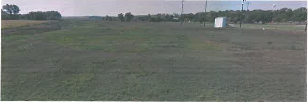
Figure 64. Clarkson Flood Control Project in Colfax County, Nebraska
