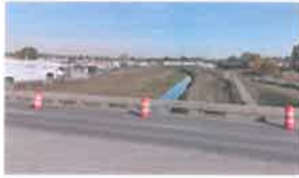
At "L" Street looking upstream
