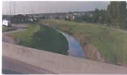
At Interstate 80 looking upstream
