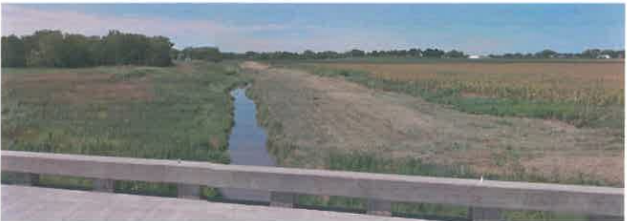
Figure 80. Highway 81 Bridge looking upstream
