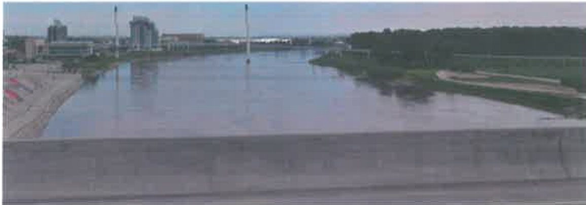
The Missouri River at the I-480 Bridge looking upstream
