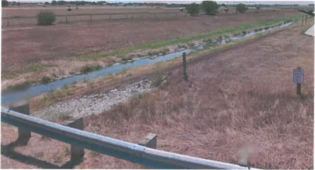
Figure 71. Lost Creek Parkway, looking downstream
