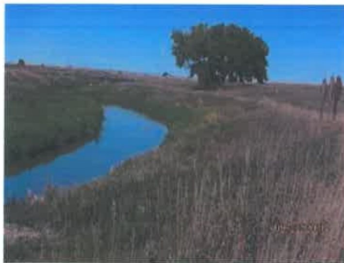
Figure 51. View of the Channel Portion of the Government Overflow Drain – Right Bank Segment near County Road P
