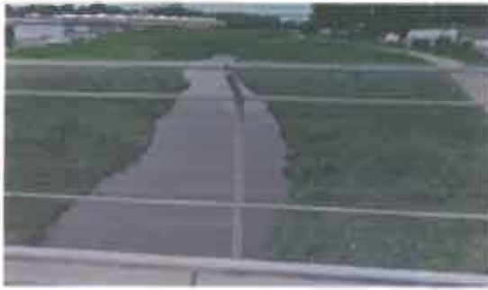
At "L" Street looking upstream
