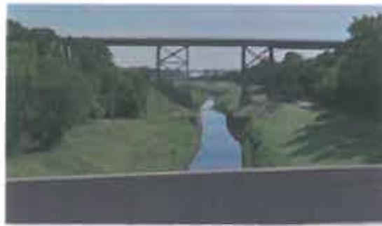
At Interstate 80 looking downstream (railroad bridge)
