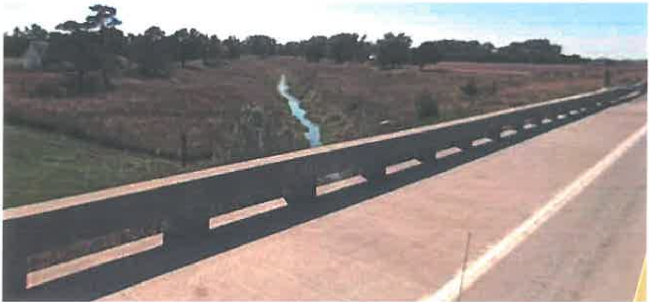
Figure 82. Front Street Bridge looking downstream
