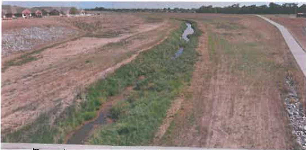
At the East Benjamin Avenue Bridge looking downstream
