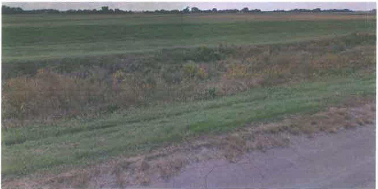
Figure 90. Highway 91 looking southwest at the levee
