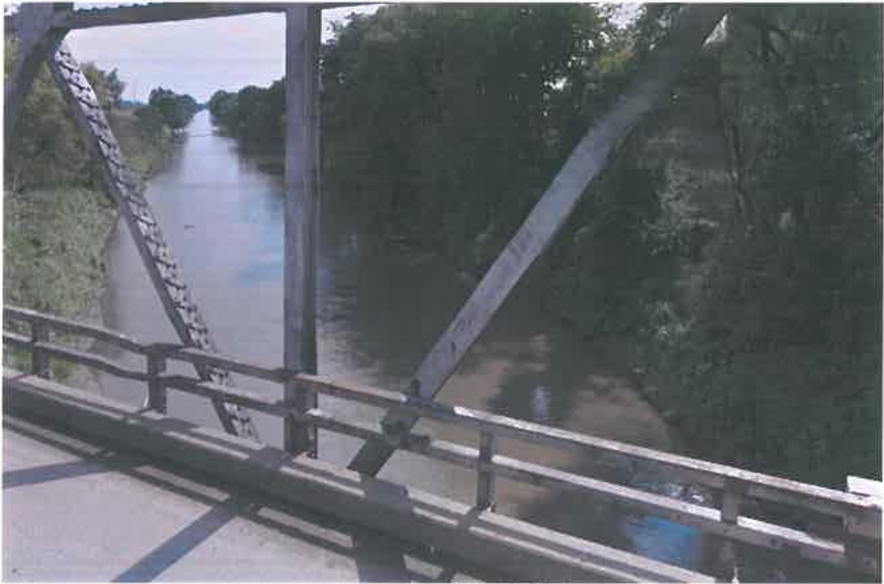
Figure 69. Pender Main Street Bridge looking downstream
