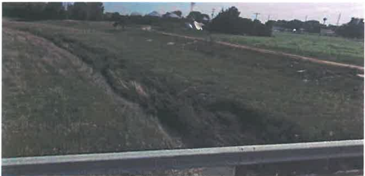
Figure 83. 4 th Avenue Bridge looking downstream
