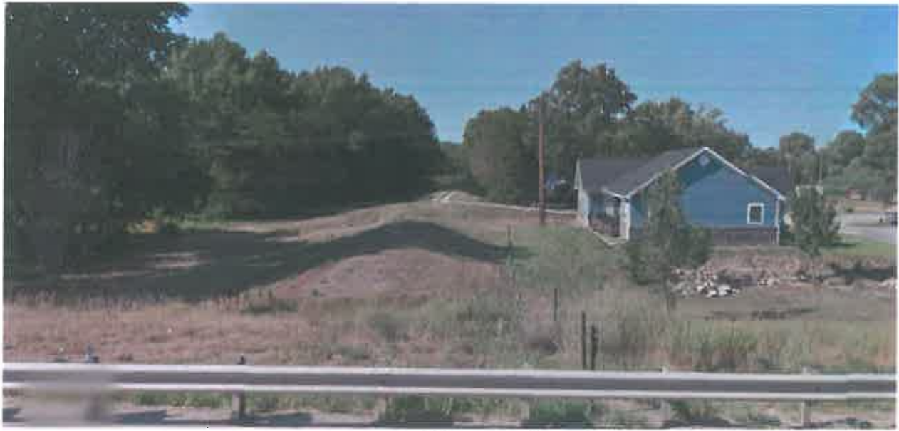
Figure 61. West Point Flood Control Project in Cuming County, Nebraska
