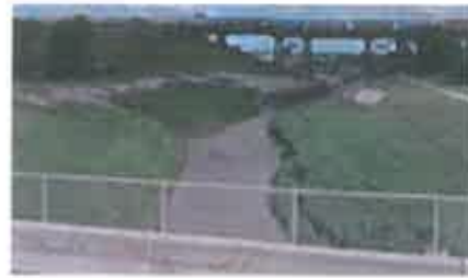
At "F" Street looking upstream
