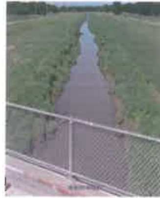
At Interstate 80 looking upstream
