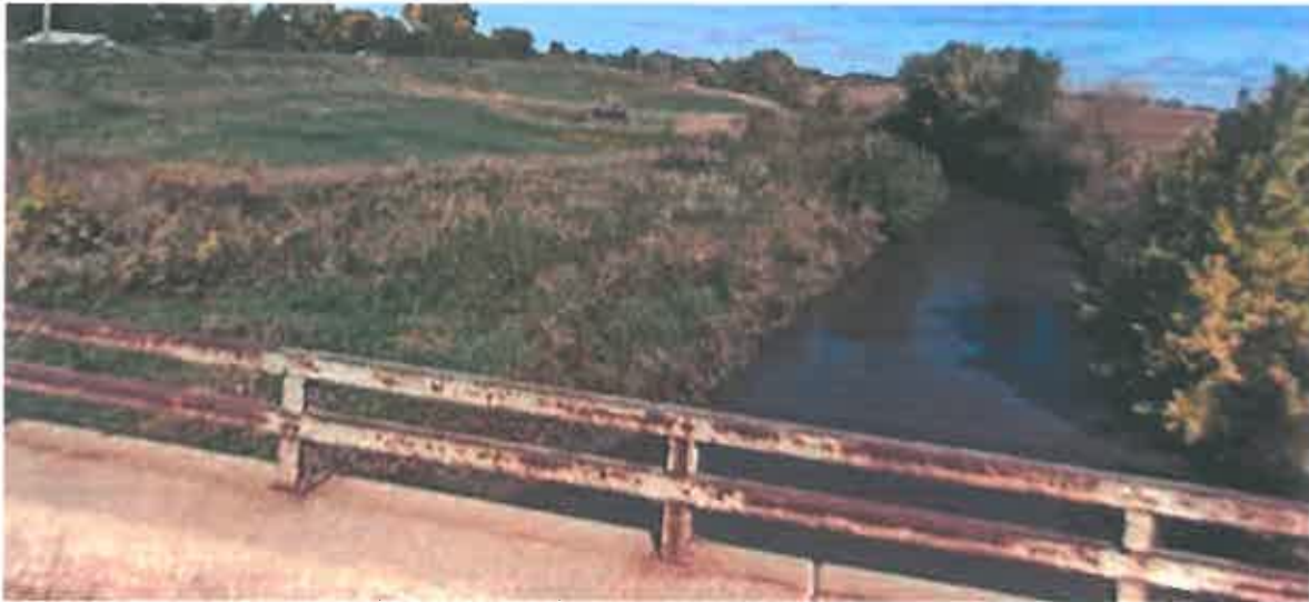
Figure 54. East Main Street Bridge looking upstream
