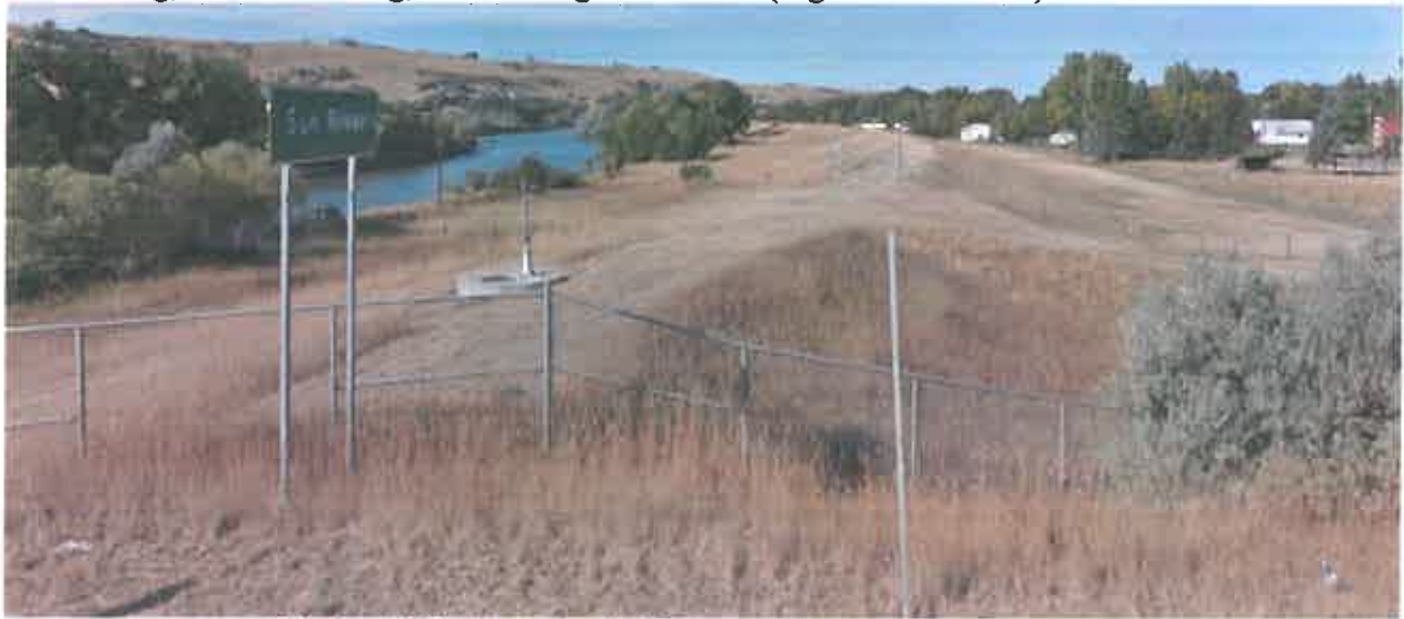
Figure 33. Great Falls Levee along the Sun River as seen from the Interstate 15 Bridge
