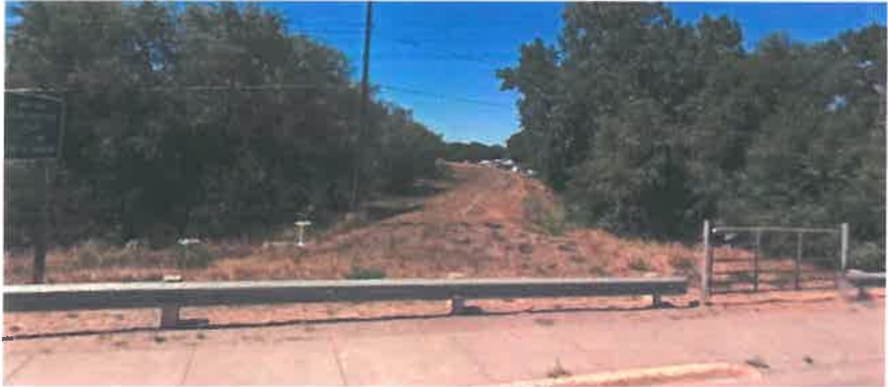
Figure 29. Havre Levee as seen from the 7th Avenue North Bridge (Left Bank)
