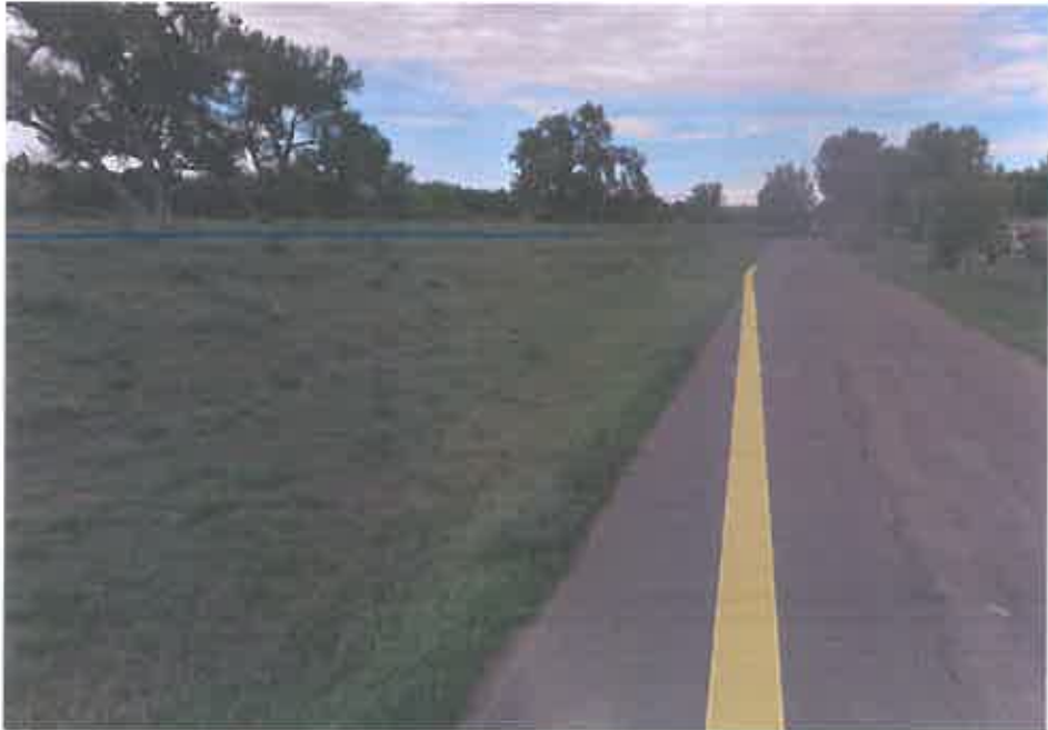
Figure 18. Forsyth Levee (Blue Line) as seen from Oak Street and 1st Avenue West
