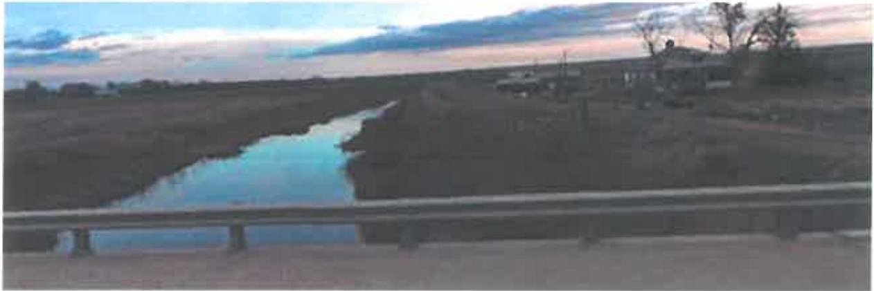
Figure 39. Saco Levee adjacent to Beaver Creek as seen from the U.S. Route 2 Bridge
