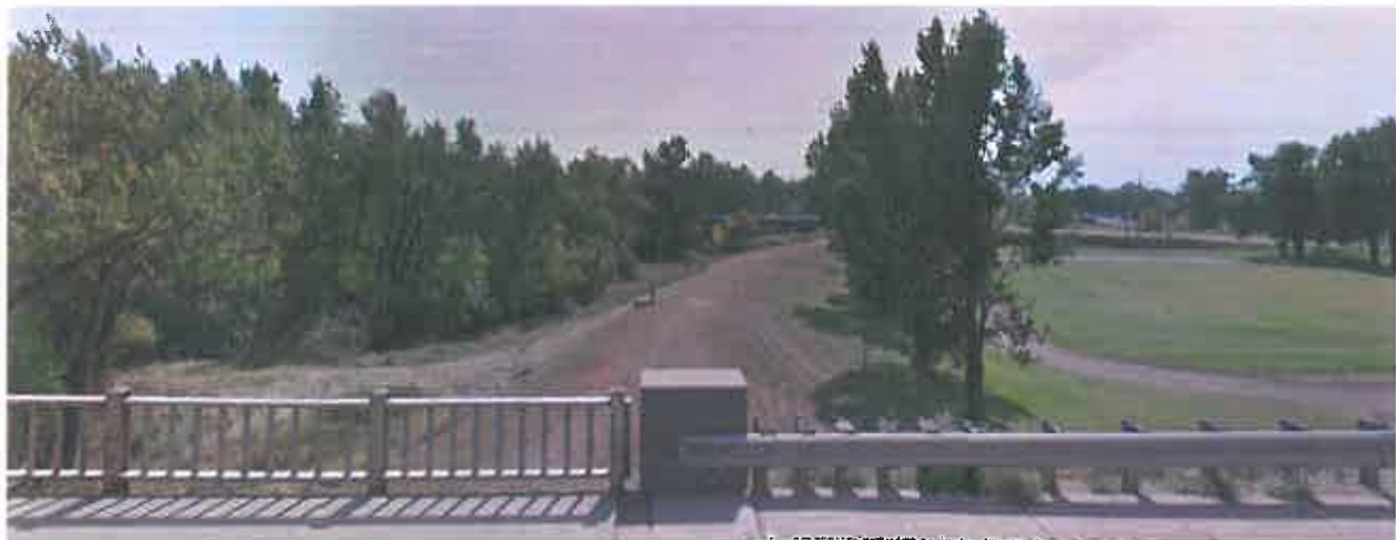
Figure 22. Typical View of the West Glendive Levee as seen from Highway 94
