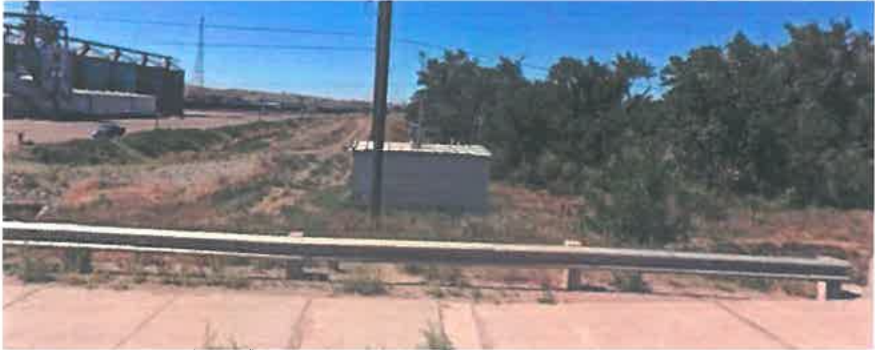
Figure 31. Havre Levee as seen from the 7th Avenue North Bridge (Right Bank)
