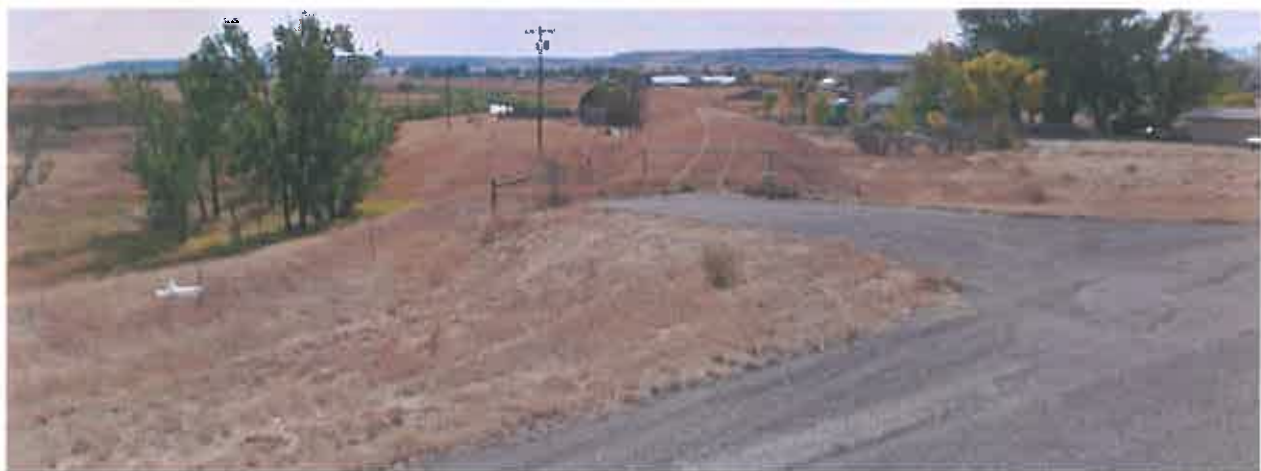
Figure 36. Vaughn Levee as seen from U.S. Highway 89
