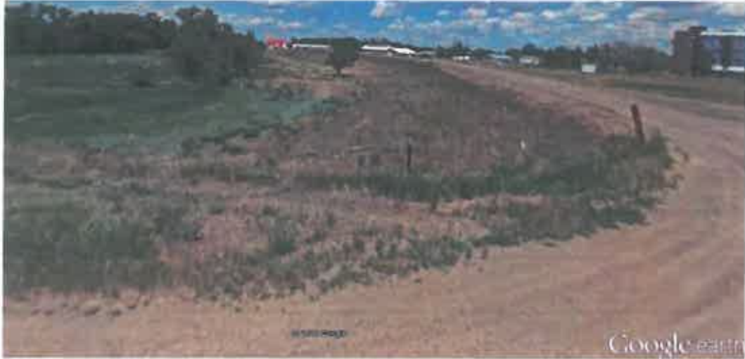
Figure 25. Typical Glasgow Levee Conditions as seen from 6th Avenue
