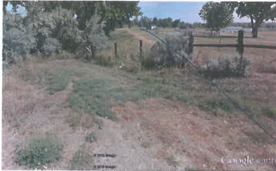
Figure 19. Forsyth Levee (Blue Line) as seen from 15th Avenue
