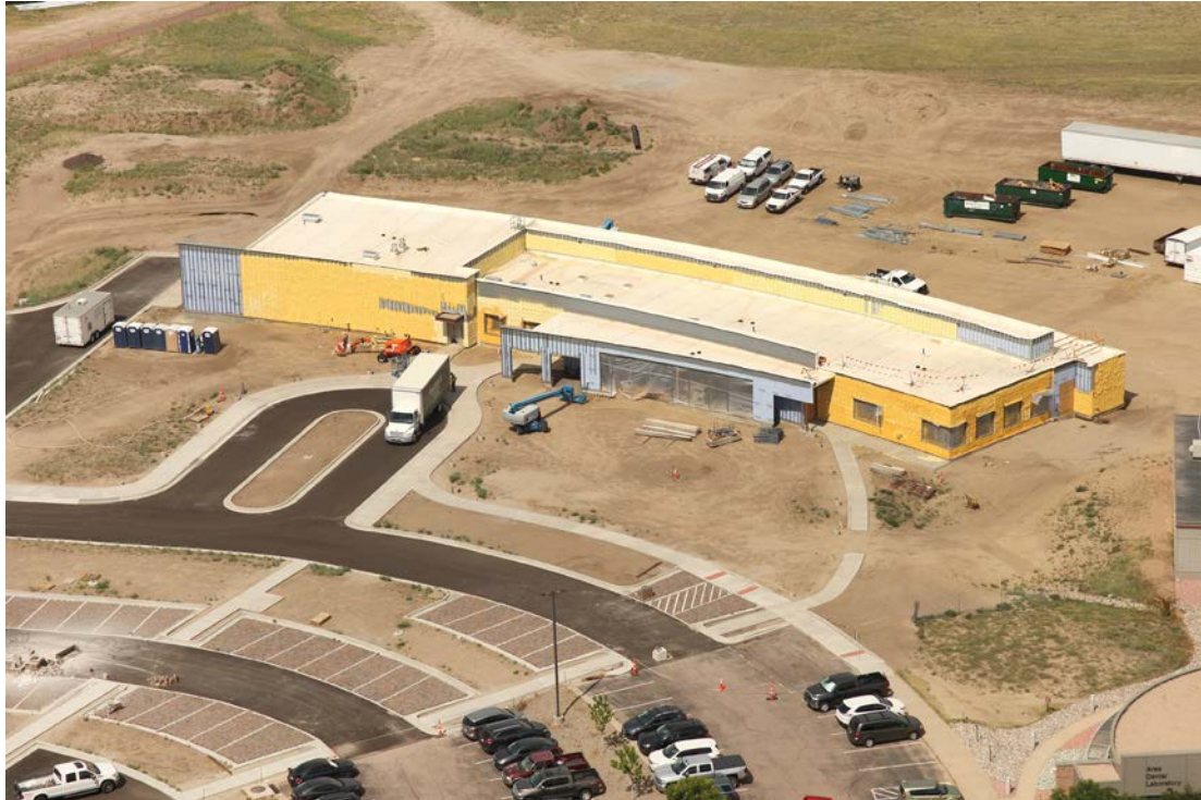
The final touches are being put on a new dental clinic on Peterson Air Force Base, Colorado. The U.S. Army Corps of Engineers, Omaha District, is building the for the 21 st Space Wing, Dental Detachment, to provide dental readiness for not just Airmen located in the area but for all military members from the greater Colorado Springs area. (Photo by Harry Weddington, USACE Photographer)
