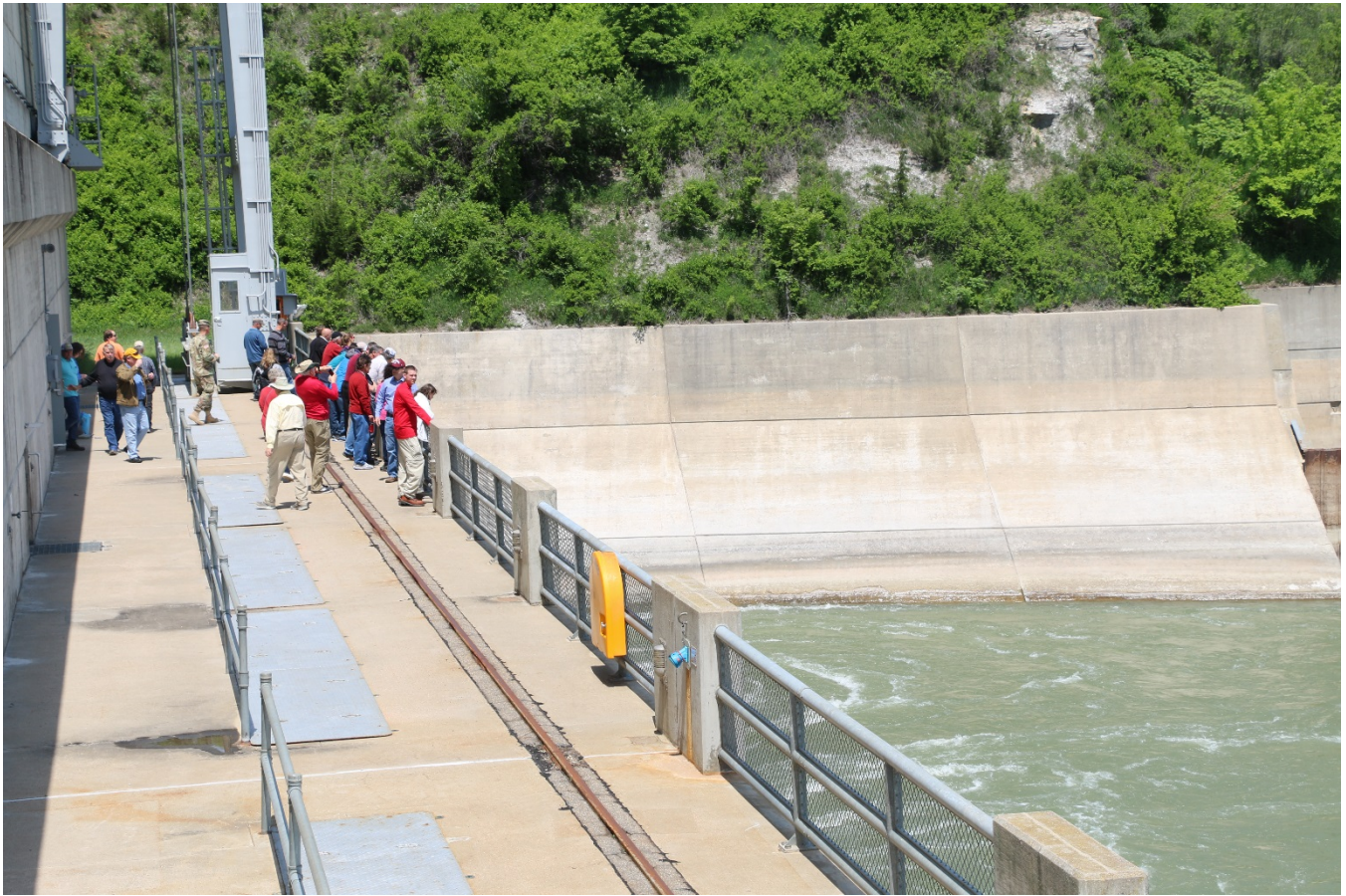
Members and support staff of the Missouri River Recovery Implementation Committee visited the Gavins Point Dam to learn more about the dam's operations and facilities as part of their May 22 field trip. (Photo by Capt. Ryan Hignight)
